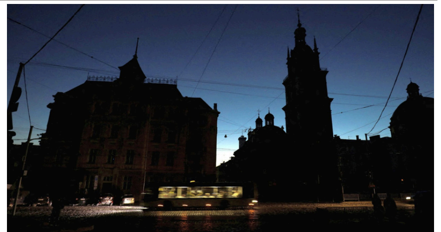
Ukraine was scrambling to turn lights and heating back on after Russian attacks targeting energy infrastructure had crippled some of the country's power generation on Sunday. Moscow, which has escalated attacks on Ukraine's infrastructure in recent months, launched hundreds of drones at energy facilities across the country overnight. The Russian attacks interrupted electricity, heat and water supplies in several cities. Russia aims to freeze Ukrainians into surrender.
